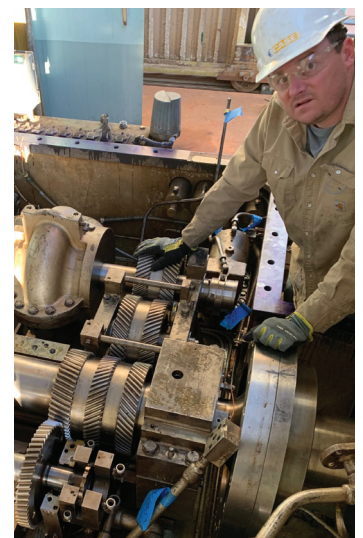
Installation inside a steam turbine front standard.
